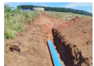
Pipelaying in progress and backfilling
