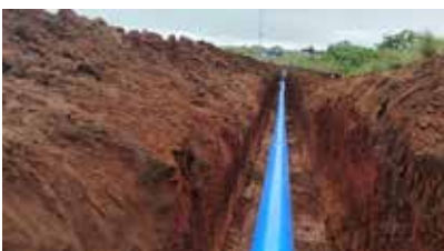
Pipe laying in progress.
