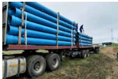
355mm OPVC pipe being delivered.
