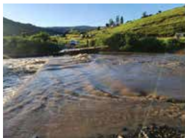
Figure 2: Dabe bridge in Ward 3 Ofafa area under Ubuhebezwe
