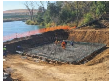
Slab for pump house
