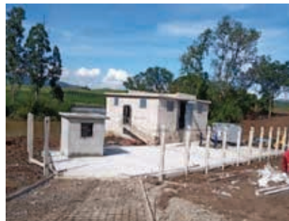
Complete pump house
