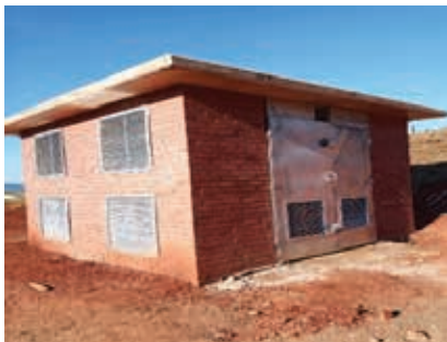
Inhlambamasoka Pump house
