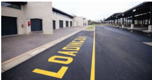
The state of the art newly built Taxi & Bus Rank in uMzimkhulu
