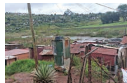
Flooding in Ixopo Fairview (shacks built on the riverbank)
