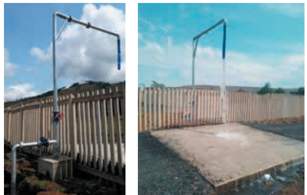
Completion and operation of Tanker Filling Station – final snagging underway.
