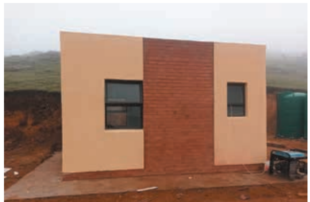
Completed Guardhouse at the Package Plant Site
