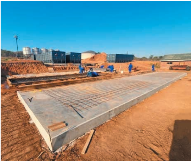
Civil Works - Preparation for sand filters platform
