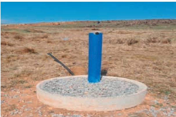
Completed Standpipe at Mpumulwane Village
