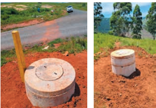
Completed valves on RM2 Pipeline.
