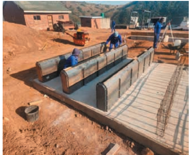
Tank Slab Plinths in progress
