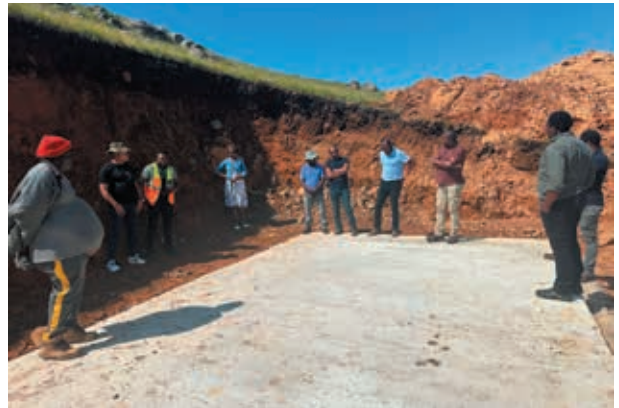
Slab Construction for the Package Plant for the Khukhulela Water Scheme
