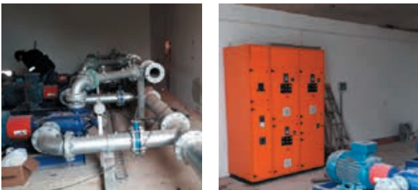
Booster PS – final completion snagging works underway.
