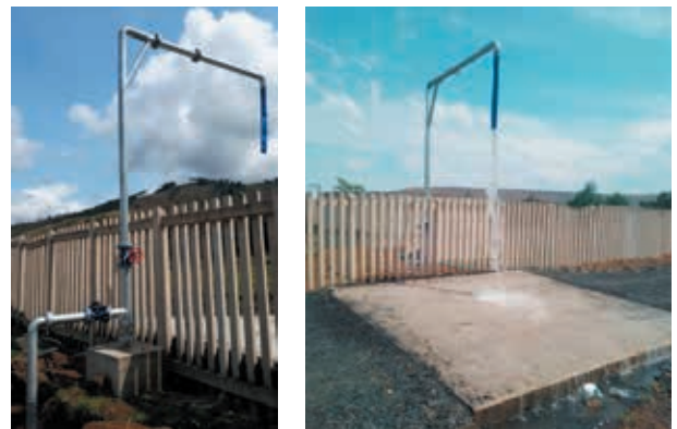
Ukuqedelwa nokusebenza kwendawo yokwetha amaloli amanzi – isigaba sokugcina nokubheka lapha nalapha okuqhutshwayo manje.
