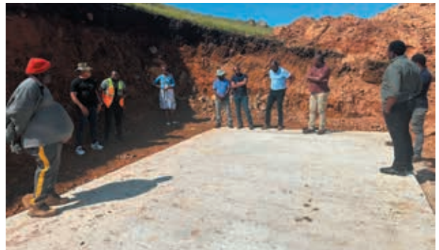
Ukwakhiwa kwesilephu sePackage Plant kohlelo lwamanzi eKhukhulela.
