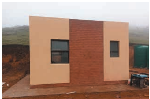
Indlu yomqaphi esiphelile ePackage Plant.
