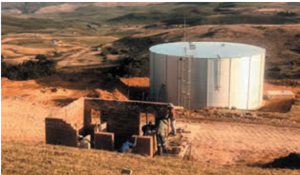
Ukwakhiwa kwendlu yomqaphi endaweni yePackage Plant nesigcinamanzo eKhukhulela.
