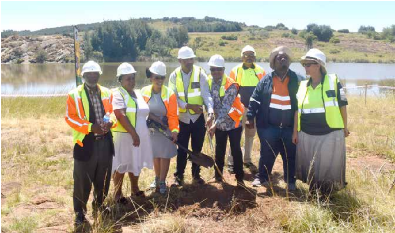
Sod turning of Raising of Kempdale Dam.
