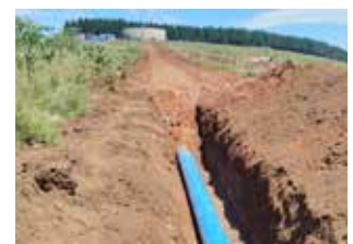
Kondlalwa imibhobho, unokhontilakhi sele ondlele i486mm yombhobho oyi355mm, lo msebenzi wenziwe ngeentsuku ezinthathu ezilandelanayo
