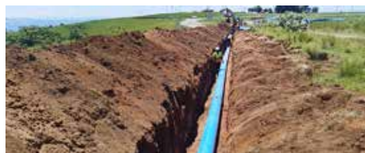
Kondlalwa imibhobho, unokhontilakhi sele ondlele i486mm yombhobho oyi355mm, lo msebenzi wenziwe ngeentsuku ezinthathu ezilandelanayo
