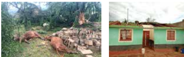
Figure 1 & 2: Depicts Lightning incident and strong wind damage occurred at Dr Nkosazana Dlamini-Zuma LM
